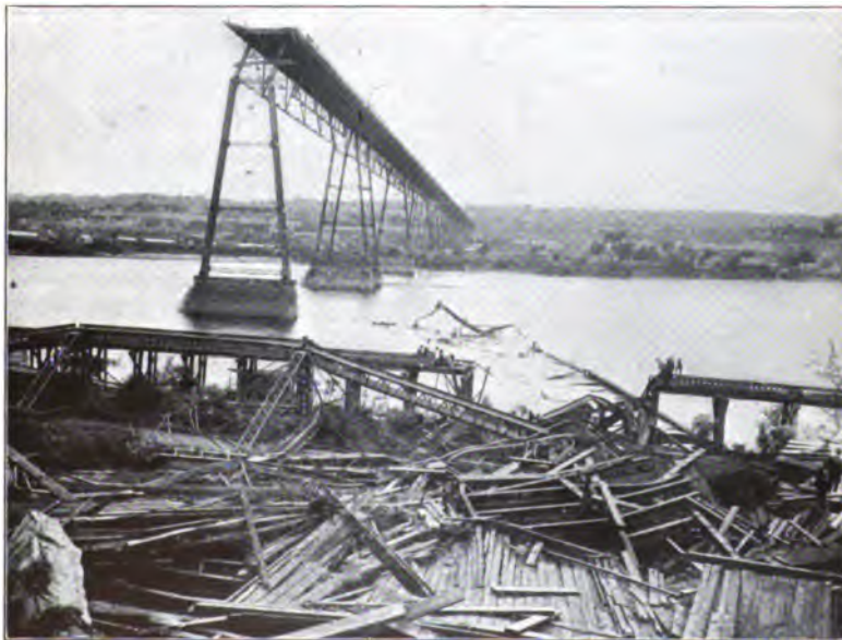
FIG. 2.—SMITH AVE. VIADUCT. VIEW LOOKING NORTHWEST
